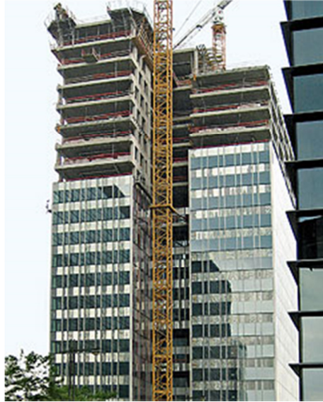
Figura 29 - Dexia Tower Building ( http://techne.pini.com.br , 2014)
